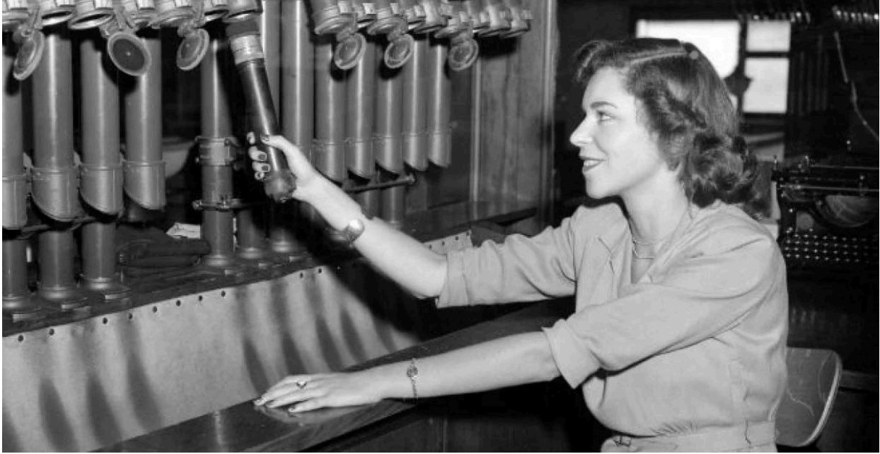
Pneumatic tube delivery system
